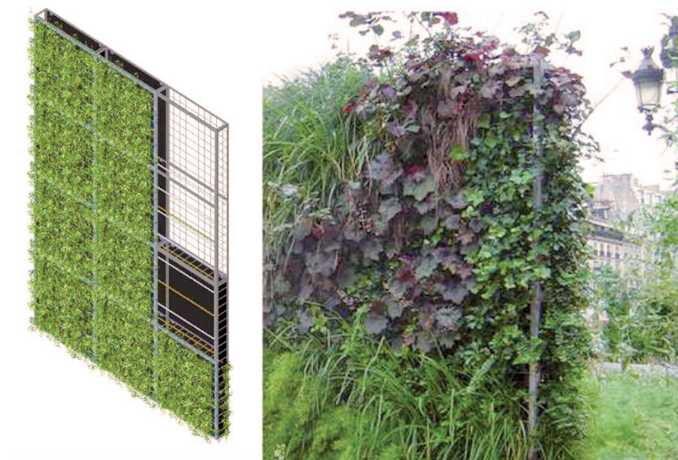
A vegetative wall: composition (left); installation (right).
