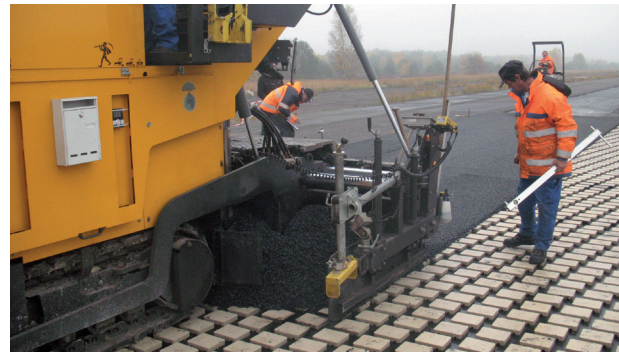
A resonator covered with porous asphalt (left) and the construction of a resonator-improved porous asphalt (right).
