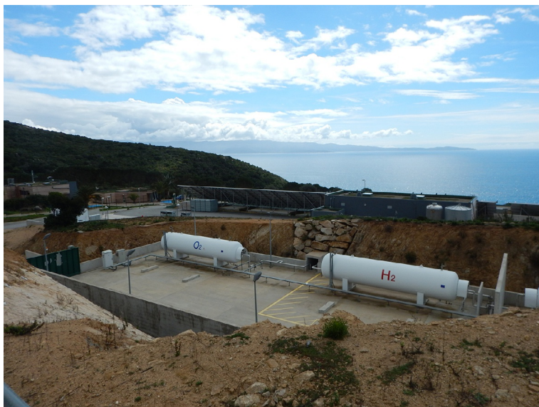
PICTURE 8.2 Burials of hydrogen and oxygen tanks (authors' pictures, April 2015).
